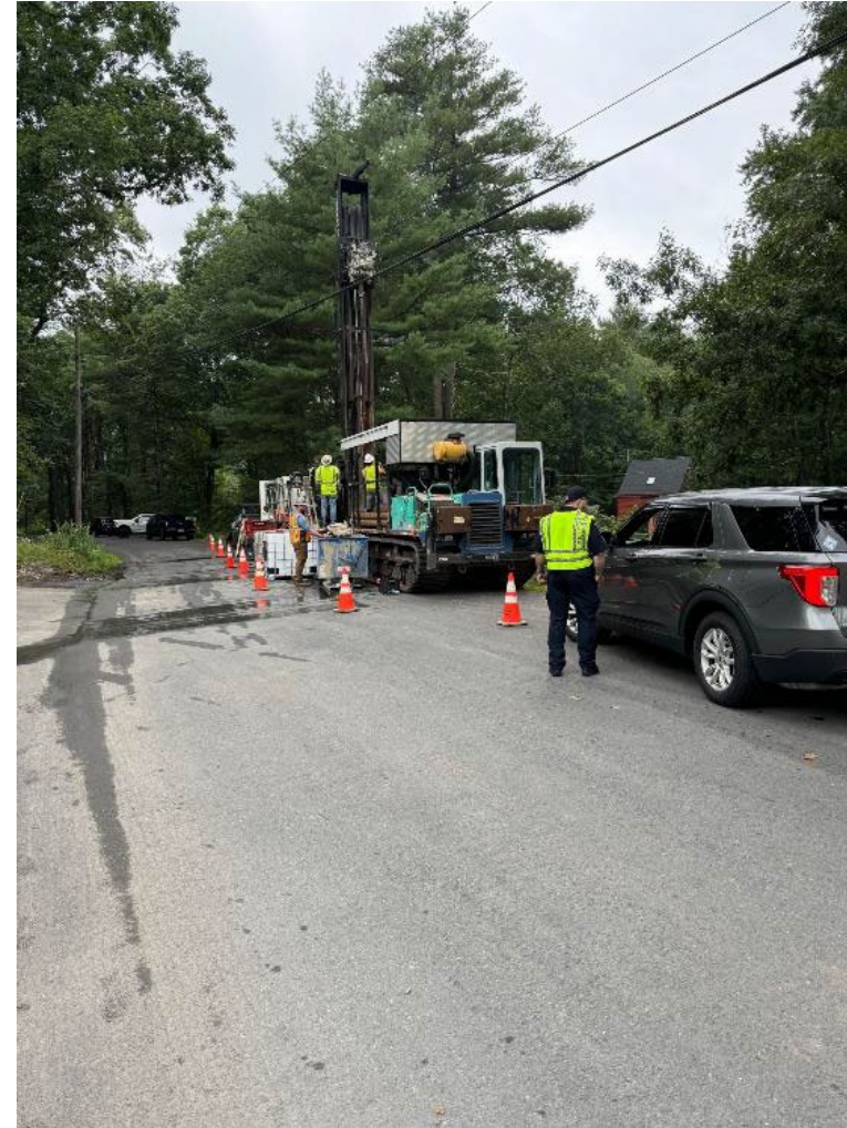
Monitoring Well Installation (Sonic Drilling)
