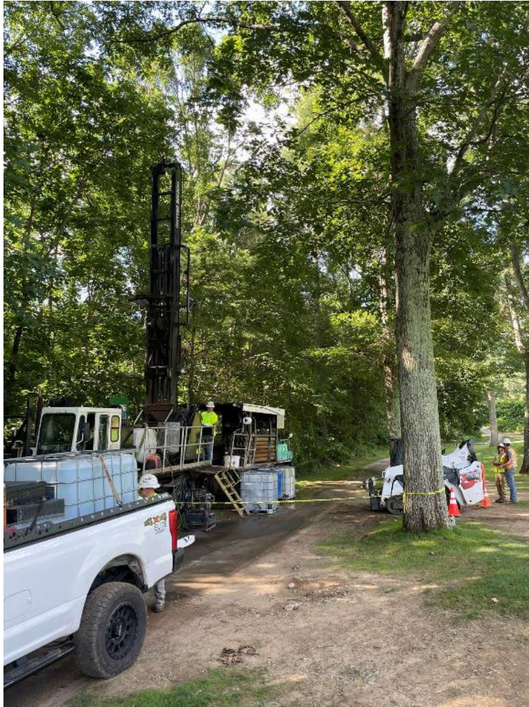
Monitoring Well Installation (Sonic Drilling)
